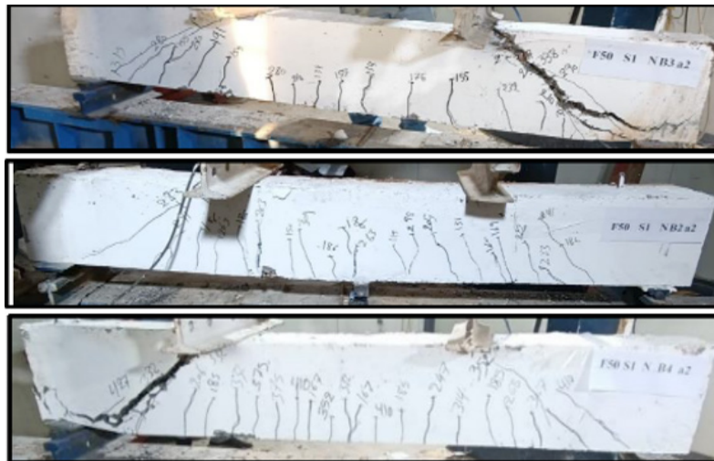
Figure 8. Crack pattern of test specimens under the effect of flexural reinforcement with steel fiber
